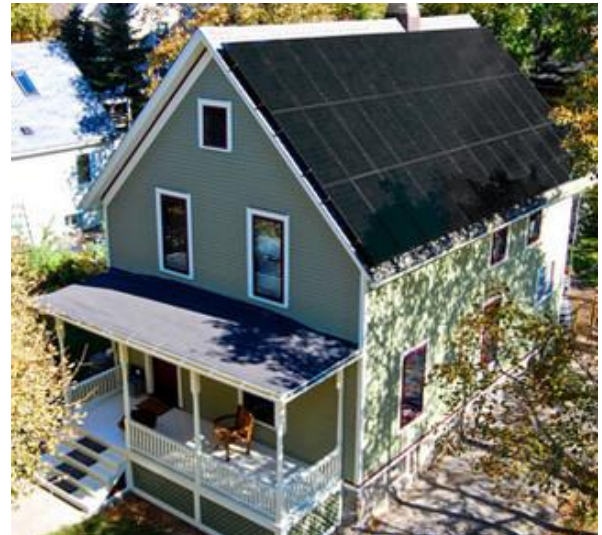
Solar panels that blend with the existing roof. Note, more expensive solar panels generally include pure black panels that do not have a metal frame or rims and only extends five inches from the roof's surface
