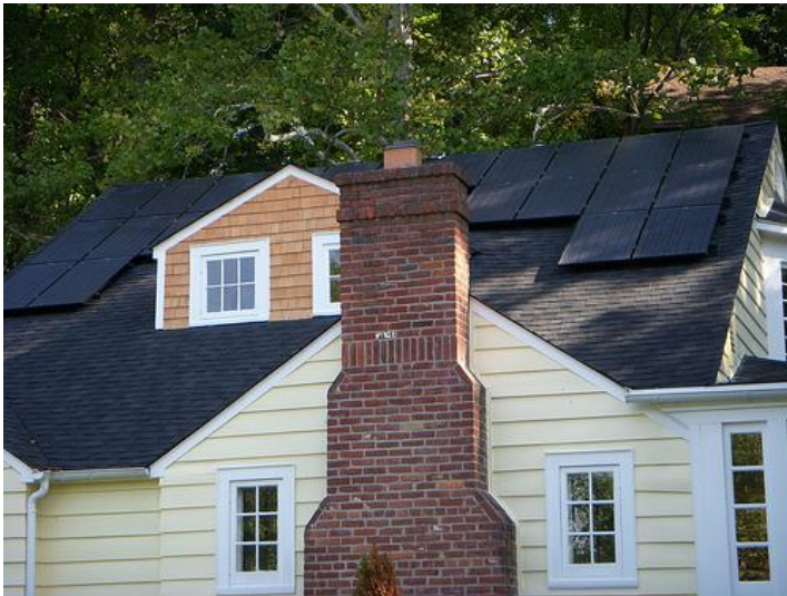
Solar panels that blend with the existing roof. Note, more expensive solar panels generally include pure black panels that do not have a metal frame or rims and only extends five inches from the roof's surface
